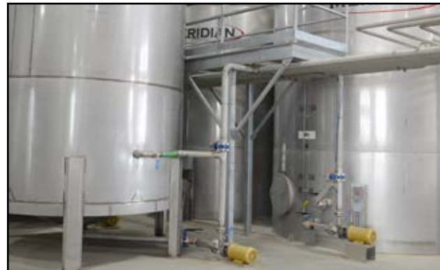
Fig 20 - Permanent fill and discharge system
