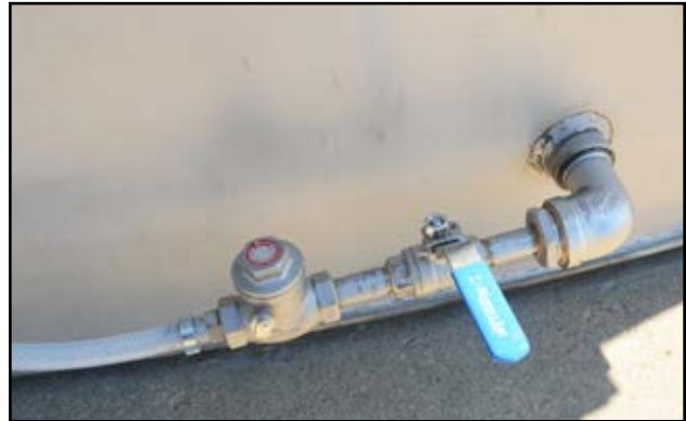
Fig 14 - Air intake pipe with valve
