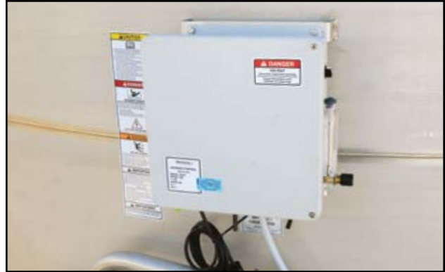
Fig 13 - Airmix liquid fluidizer control box
