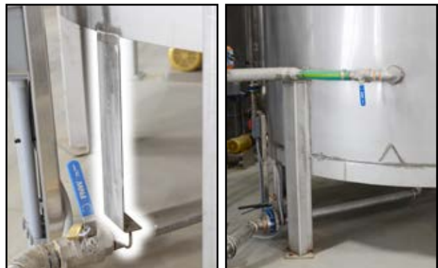
Fig 8 - Bracket to support piping from bottom coupler
