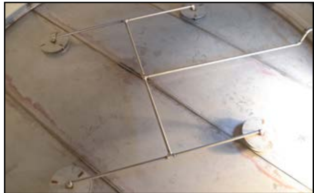
Fig 15 - Air injection diffusers
